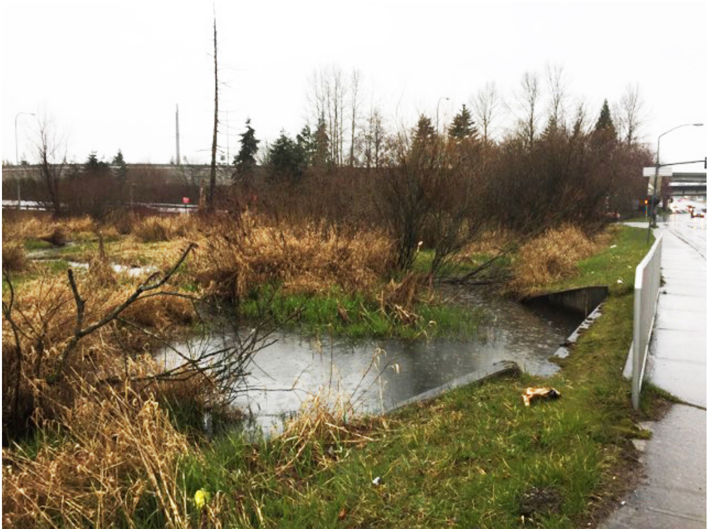
Culvert at 44th Avenue W
